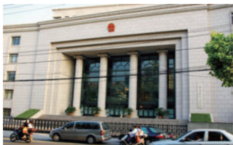
The Solution for Local Government Charging Project
